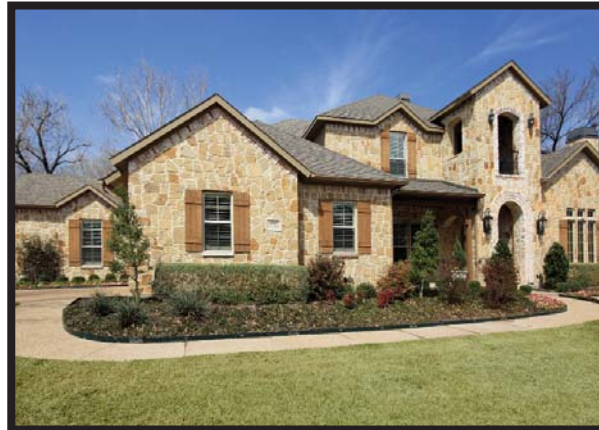
8507 San Leandro Drive
