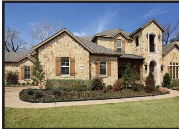
8507 San Leandro Drive
